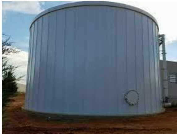
Figure 6 – example of sprinkler tank external appearance
