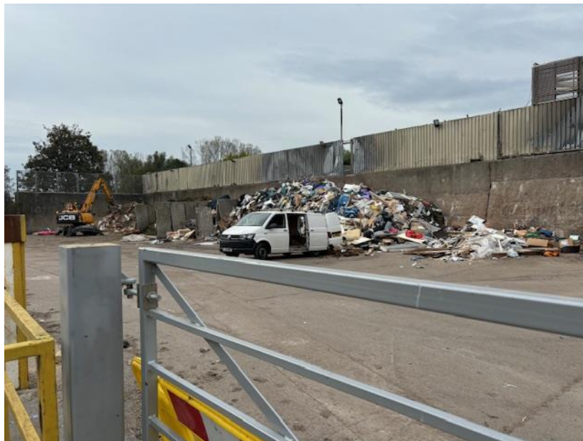
Figure 12 – existing push walls
